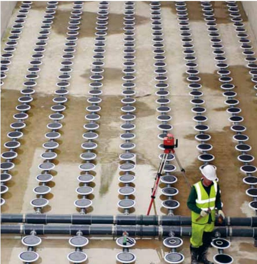
Under the right conditions, nature is the most cost-effective catalyst you can employ for wastewater treatment. Providing perfect conditions for nature to work in a man-made environment with controlled processes requires coordination of technology and biology. We have the knowledge and experience required.
